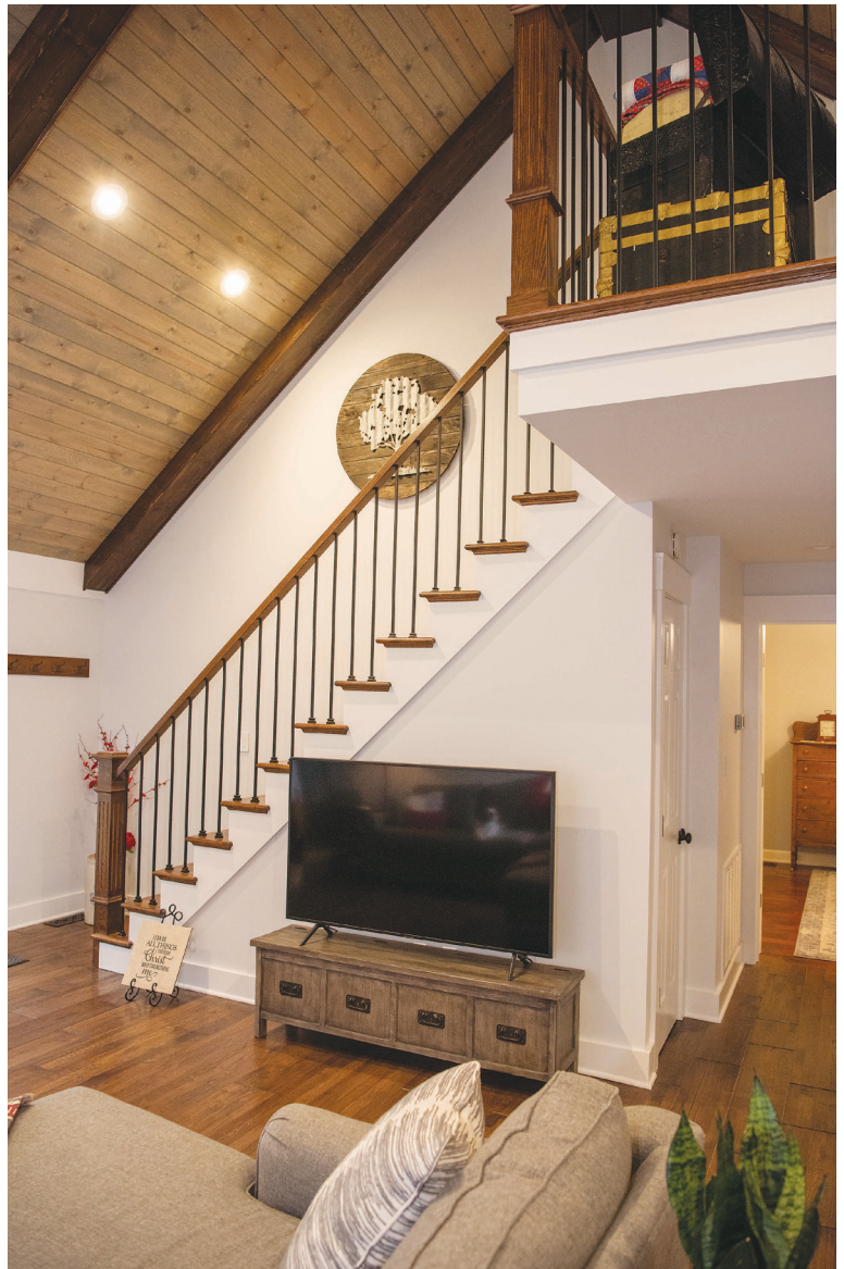
ABOVE: The room came down to the studs. The staircase was shifted flush against the back wall. Carpeting was removed and the entire space was polished and put right.
